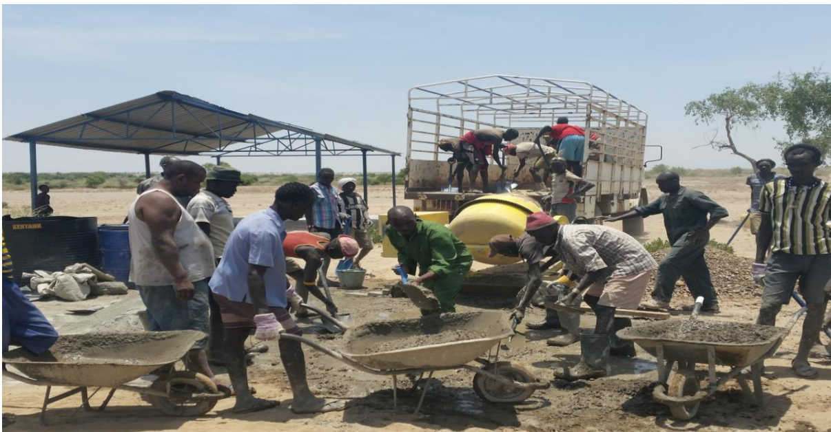
Renting a local truck is essential to collect gravel and hardcore.
