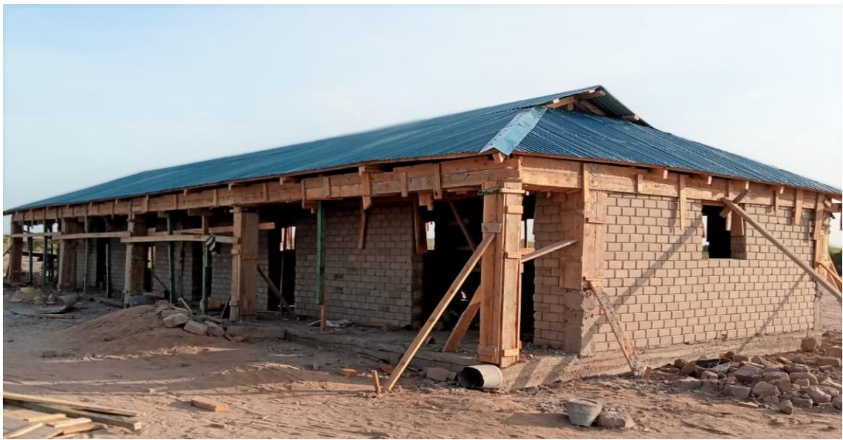
El Bokoch Teachers accommodation nearing the finishing stages
